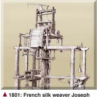
Marie Jacquard patented a loom which used punch cards to control a sequence of operations, enabling the weaving of intricate patterns
